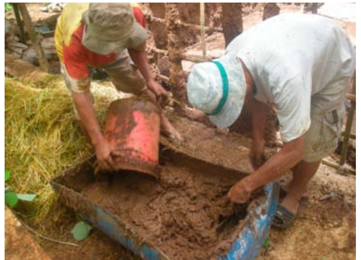
Clay, sand and water are placed/mixed in half drum
