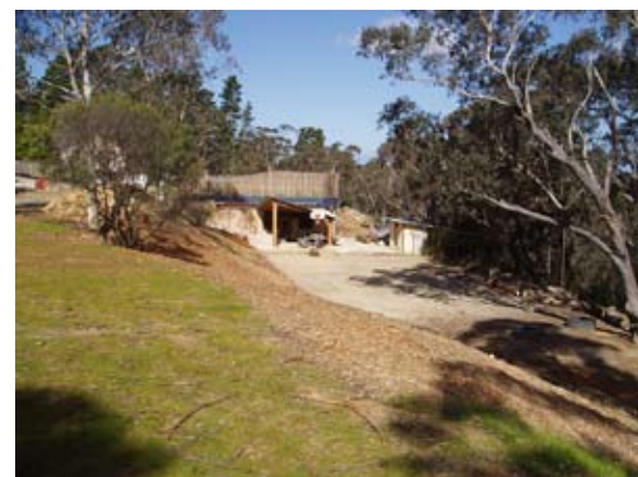
Photo 8: Roof top garden above the volunteers living quarters.
