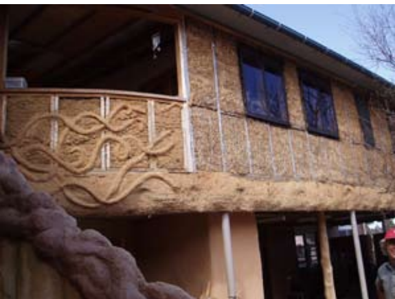
Photo 2: Straw bale wall ready for rendering.
