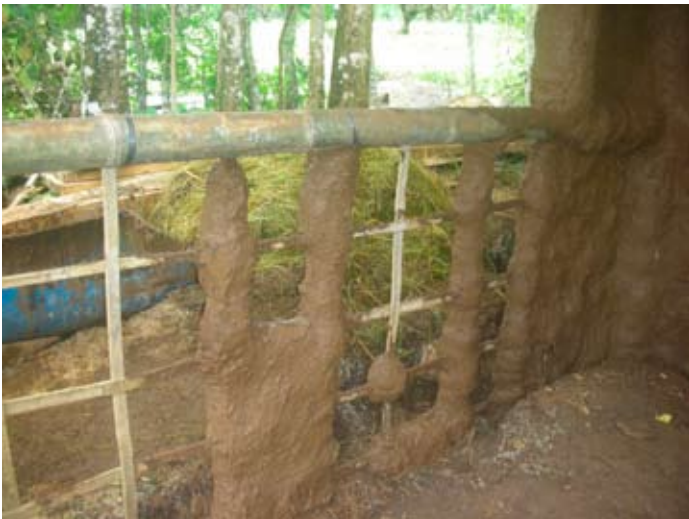
remaining space is filled with cob
