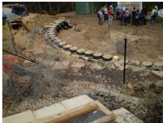
Photo 12: Old tyres and fill used to create a large retaining wall.
