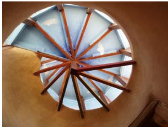
Photo 3: Internal view looking up into the spiral.
