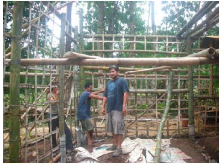
Bamboo structural frame posts to have well detailed base for moisture and termite/insect control, and structural connection.
