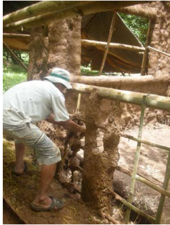
... and then tied around bamboo frame/lattice
