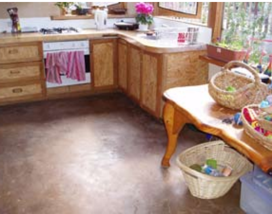
Photo 4: Earth floor of a classroom.
