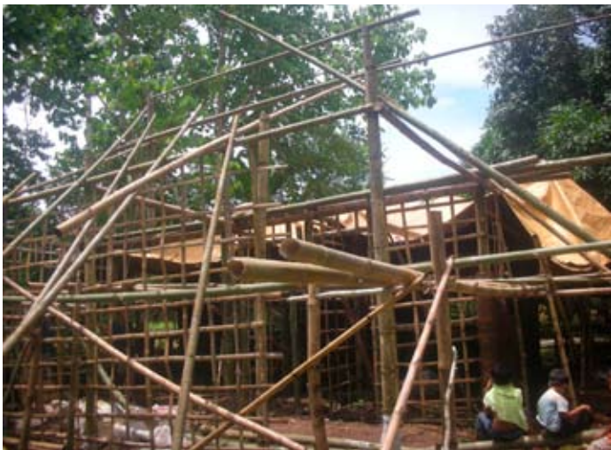
Bamboo structural frame to have adequate bracing
