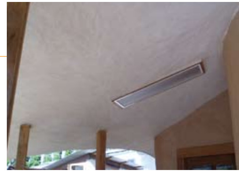
Photo 13: Mud ceiling formed over wire mesh.
