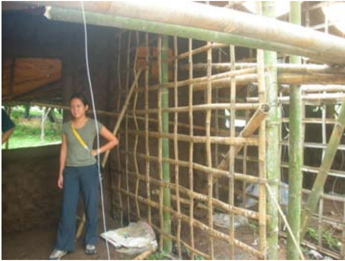
Bamboo structural frame with split bamboo woven infill
