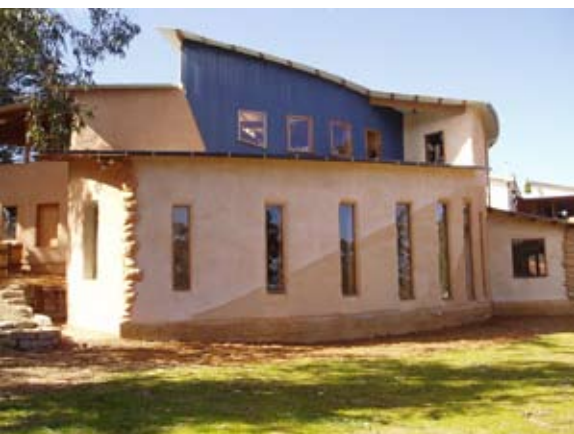
Photo 10: Southern view of main building.
