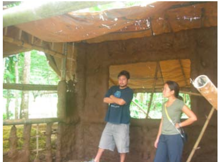
completed wall panel to right
